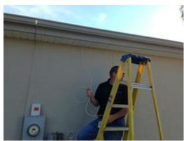
5.9 EZ Bend Cable can be fastened to masonry walls using shark tooth anchor clips³ or similar fasteners.
